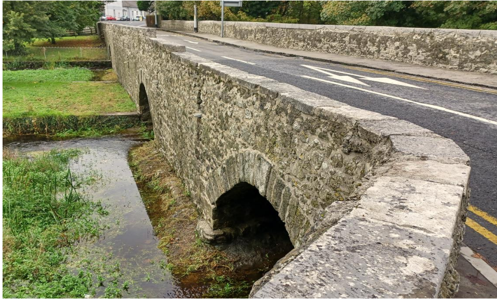
SUCK (WEST) BRIDGE, BALLINASLOE – NATIONAL MONUMENT
