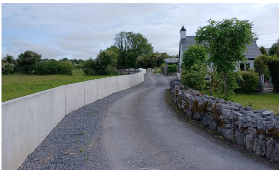
FLOOD DEFENCE WORKS COMPLETED AT PRIBBAUN, ROSCAHILL 2023
