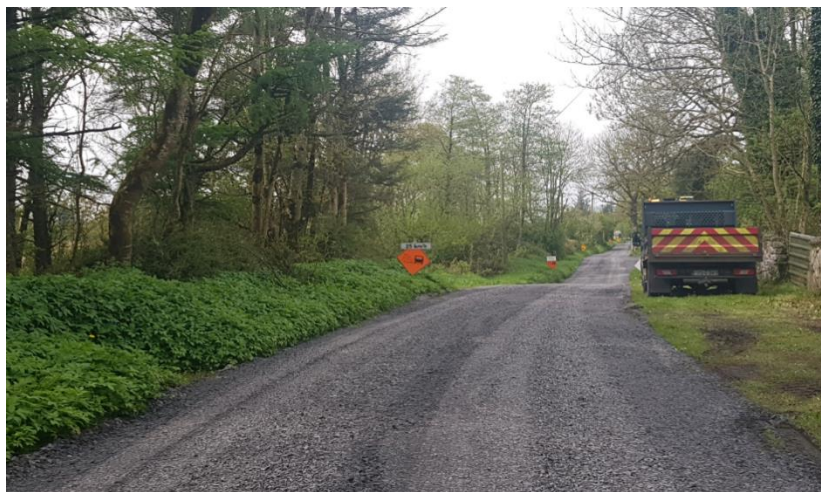
ROAD RESURFACING IN TUAM
