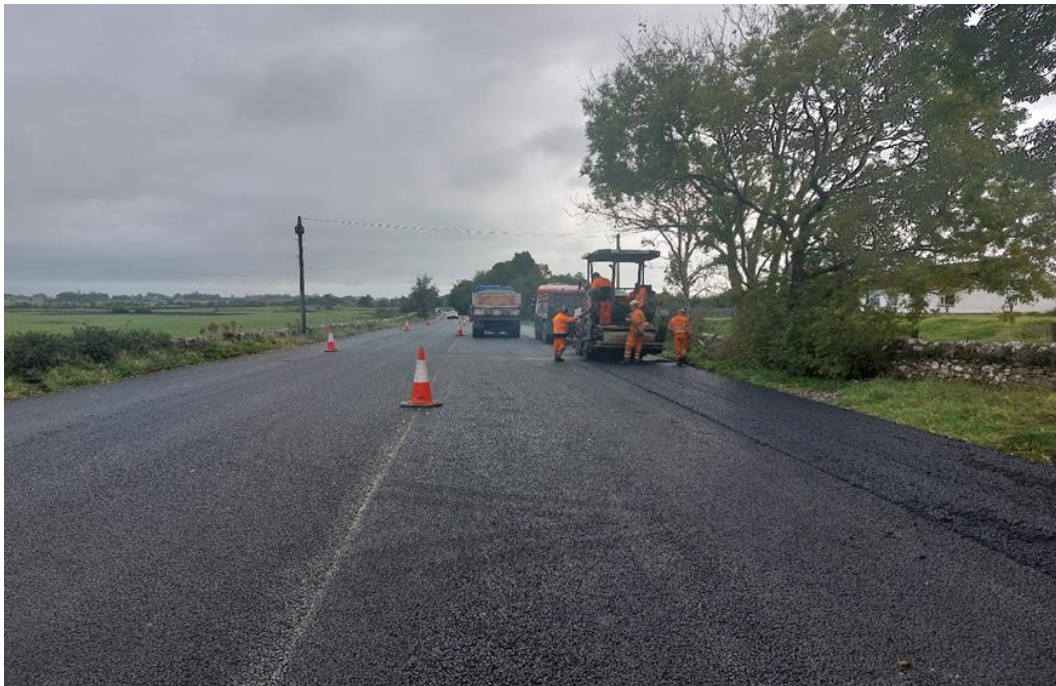
OVERLAY ON FORMER NATIONAL ROAD AT DARTFIELD, LOUGHREA – R446
