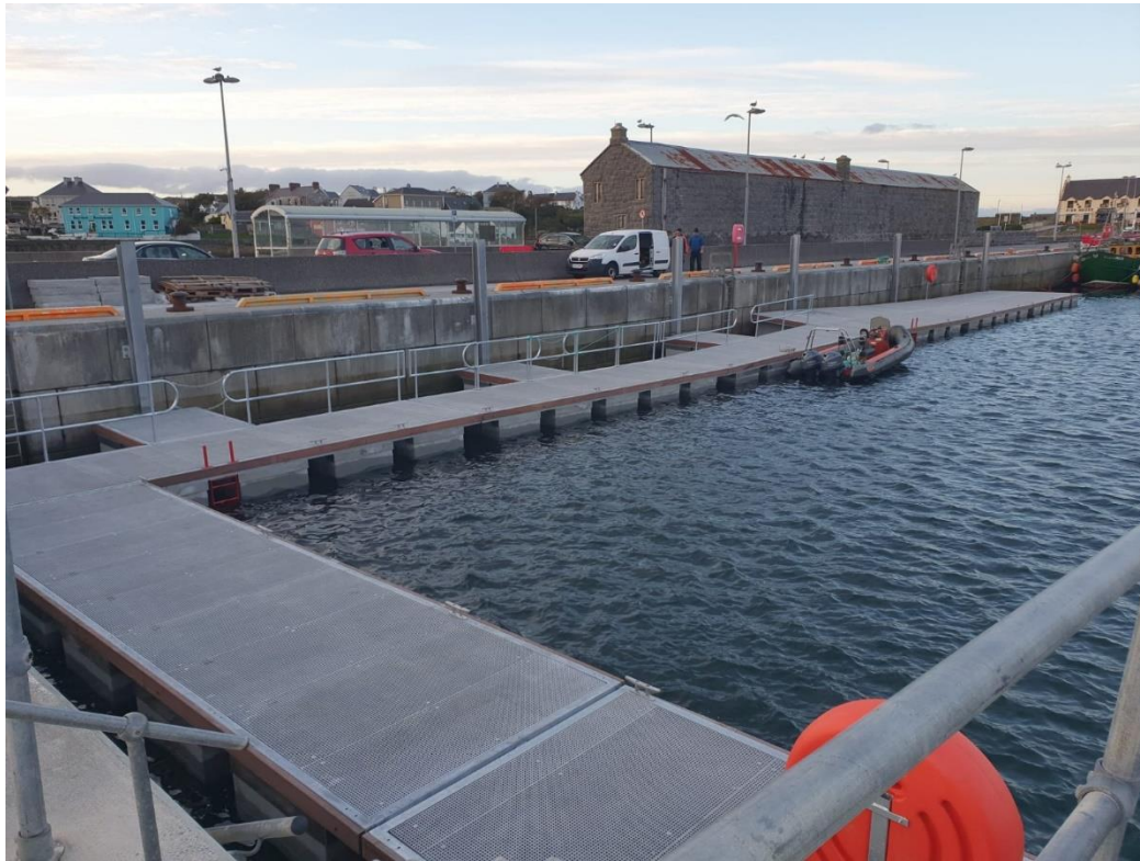
PONTOON INSTALLATION AT KILRONAN - BALAMI FUNDED PROJECT
