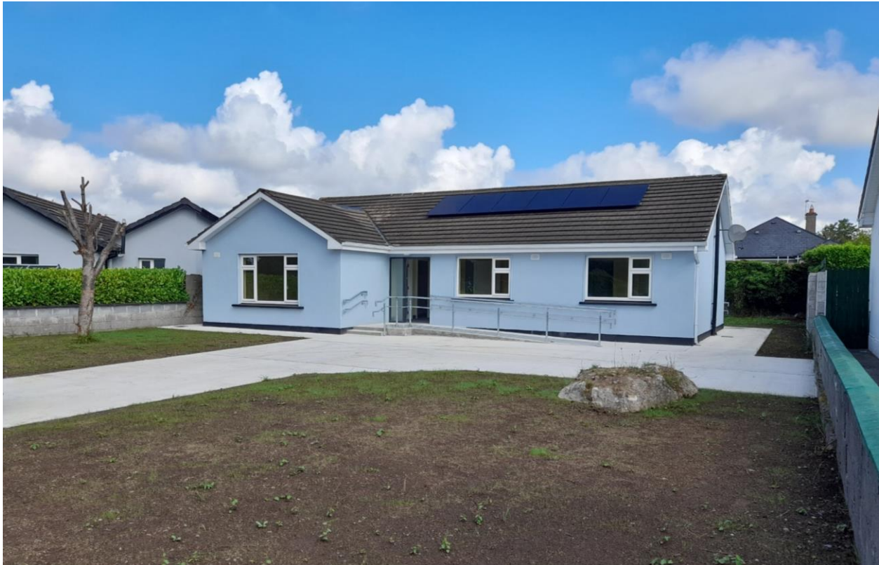
REFURBISHED AND ADAPTED TRAVELLER SPECIFIC HOUSE
