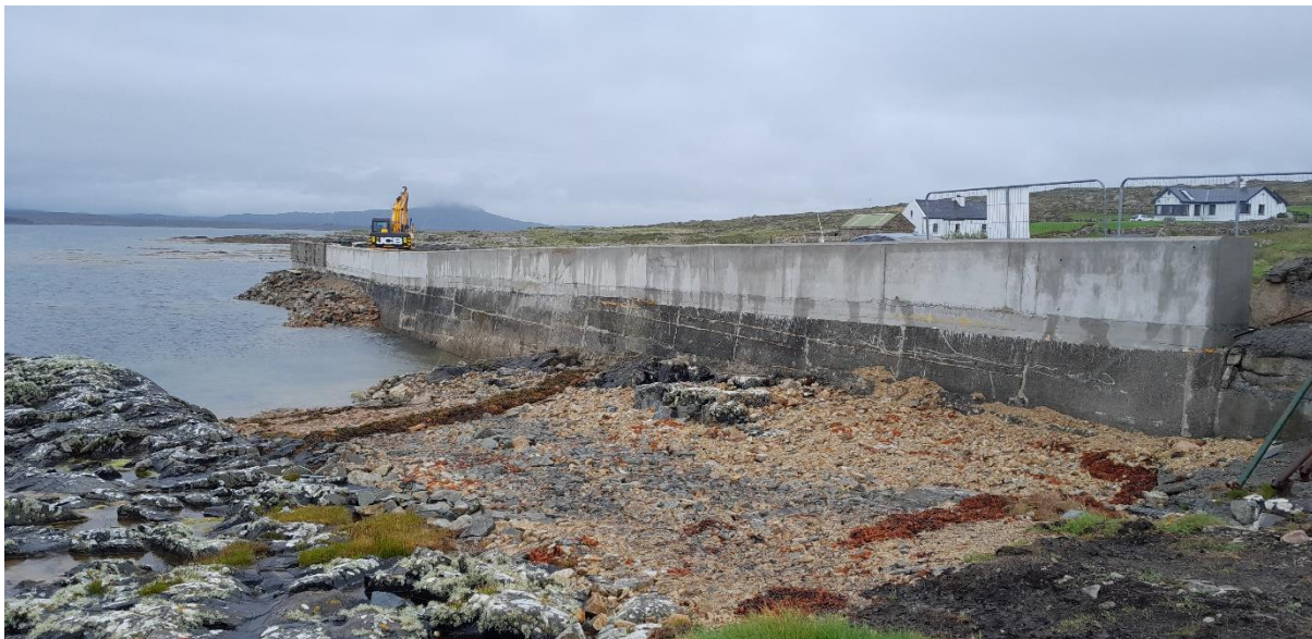
BEALCARRA STORM WALL - BALAMI FUNDED PROJECT
