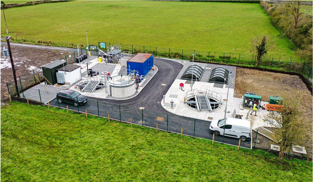
Ahascragh Wastewater Treatment Plant
