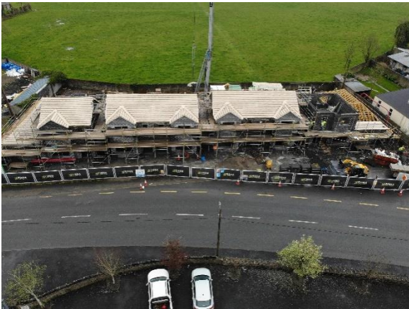
UNDER CONSTRUCTION PHOTO AT BALLYMOE MARCH 2024
